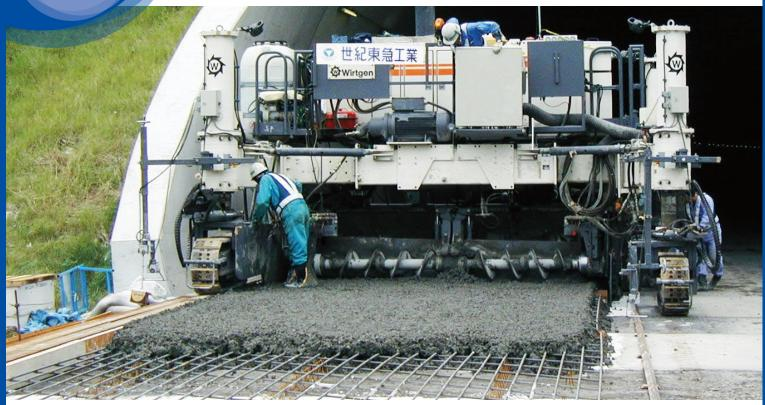
This method is to construct a concrete pavement slab without framing using special machinery.
